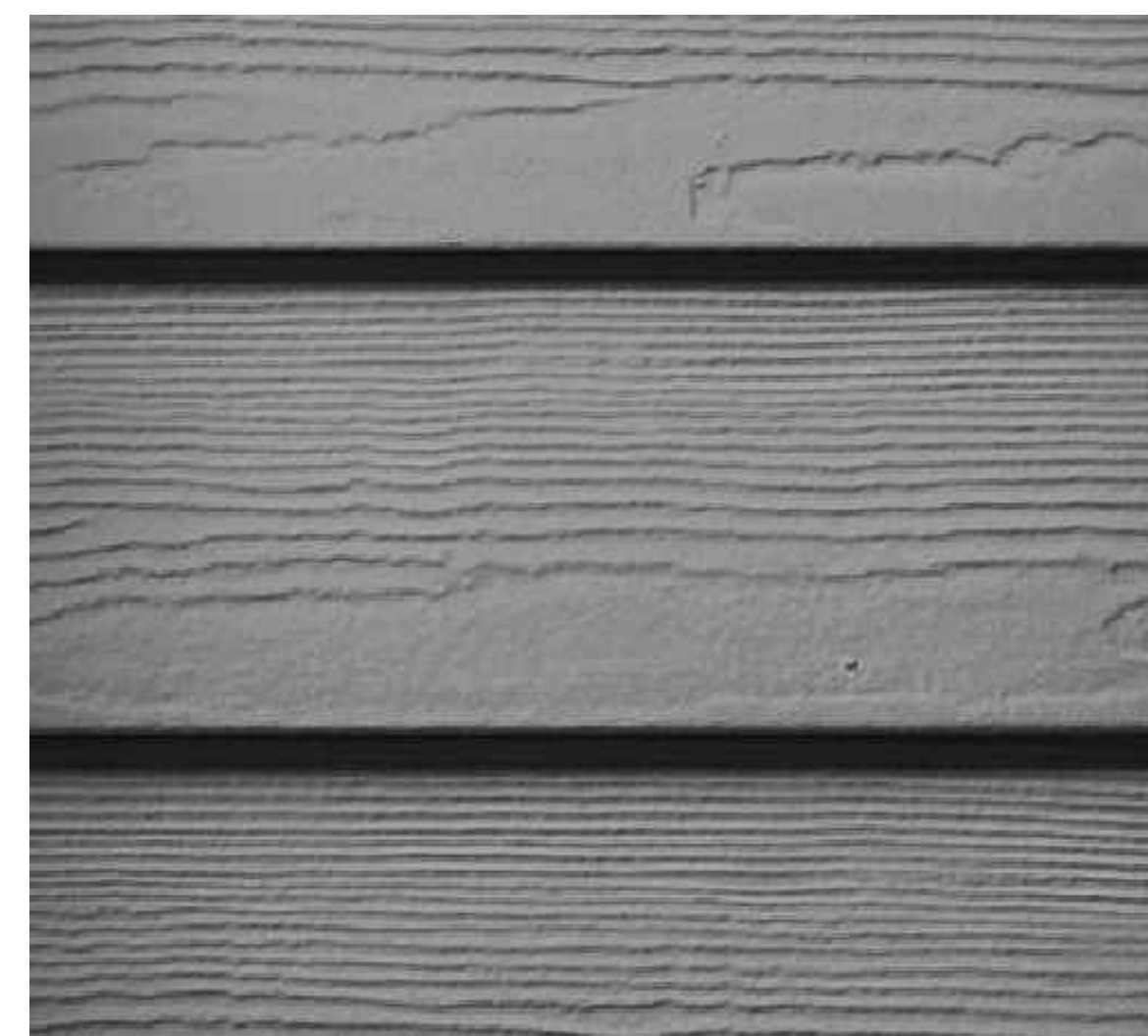
3 HORIZONTAL SYNTHETIC BOARD JAMES HARDIE OR SIMILAR
